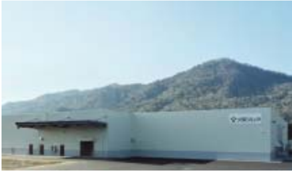
Botanical raw materials storage and processing plant
