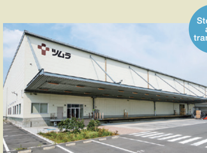
East Japan Distribution Center (storage in Kuki City, Saitama Prefecture)
