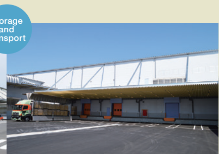
West Japan Distribution Center (Ono City, Hyogo Prefecture)
