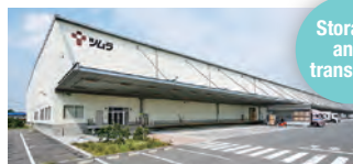
East Japan Distribution Center (Kuki City, Saitama Prefecture)
