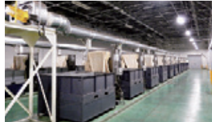
Dryer (YUBARI TSUMURA)
