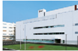
Shizuoka Plant (Fujieda, Shizuoka Prefecture)
