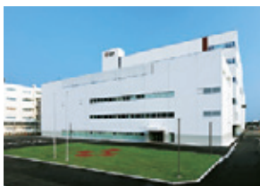
Shizuoka Plant Office and QC Building
